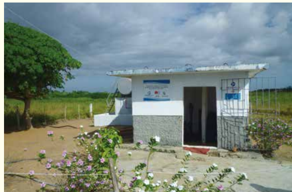
Pump station installed for “Project for Portable Water Supply System Improvement on the Isle of Youth”
