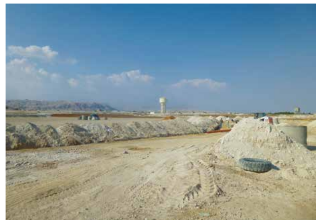
Construction of Jericho Agro Industrial Park
