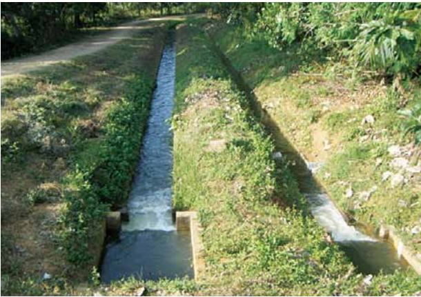
Walawe Left Bank Irrigation Upgrading and Extension Project (Dual Canal System: The left is for rice and the right is for other crops.)
